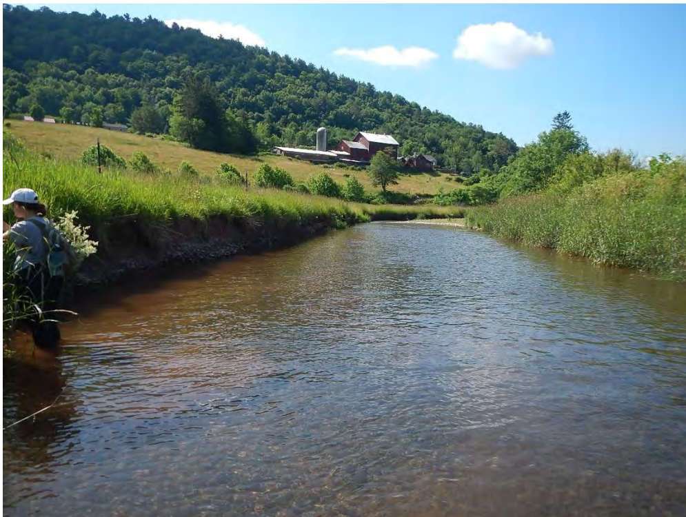
Site 9-a: Erosion along an agricultural field on the left bank. Photo taken before stabilization project was completed. Photo taken looking downstream at STA ~774+00.
